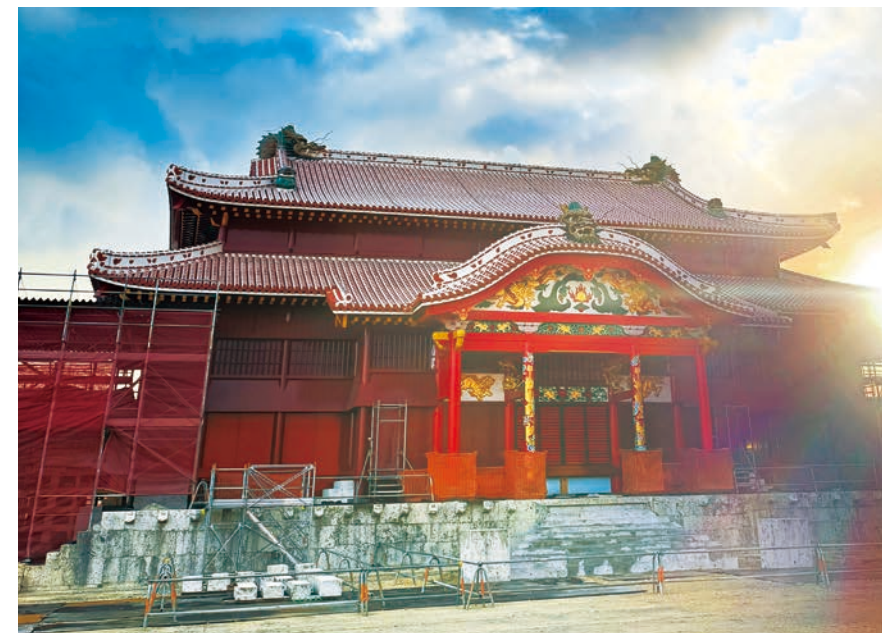
Restoration of Shuri Castle Seiden
